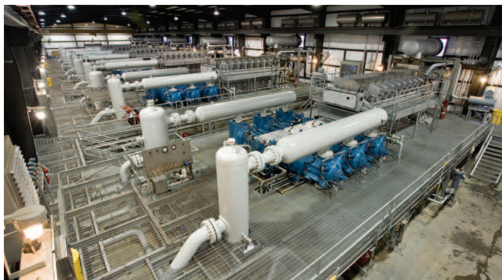
Hundreds of gas-fired electric generating and petrochemical facilities being built all across the country, along with the first wave of LNG export terminals, are ushering in a new era for the domestic natural gas market. Shown here is a row of large-horsepower reciprocating compressors in a Southern Pine Electric Power Association gas storage and transmission plant in Mississippi.
